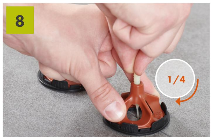
The clips are now correctly tightened and, therefore, the tiles are levelled. If the levelling is not satisfactory, additional SOS clips should be added and the clip tension should be increased by further tightening the caps.
