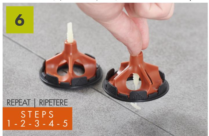
7. Now go back to the first installed SOS Rescue Clip and tension it by turning the cap by another quarter turn; keep a firm hold of the upper handle.
