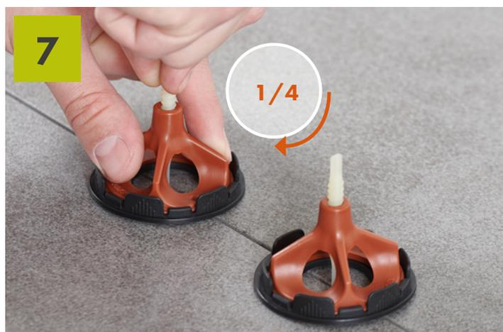
8. Now go back to the second installed SOS Rescue Clip and tension it by turning the cap by another quarter turn; keep a firm hold of the upper handle.
