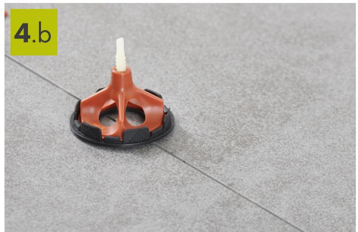
5. Tension the clip by tightening the cap by one quarter turn.
